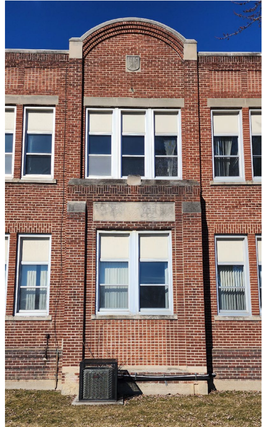
FIGURE 10 - SOUTH ENTRANCE - CENTER BAY
