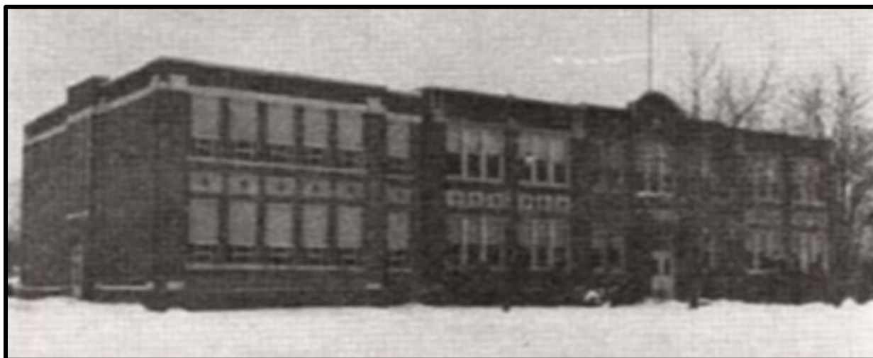
FIGURE 3 - 1951-52 ADDITION – SOURCE OFFICIAL OPENING PROGRAM
