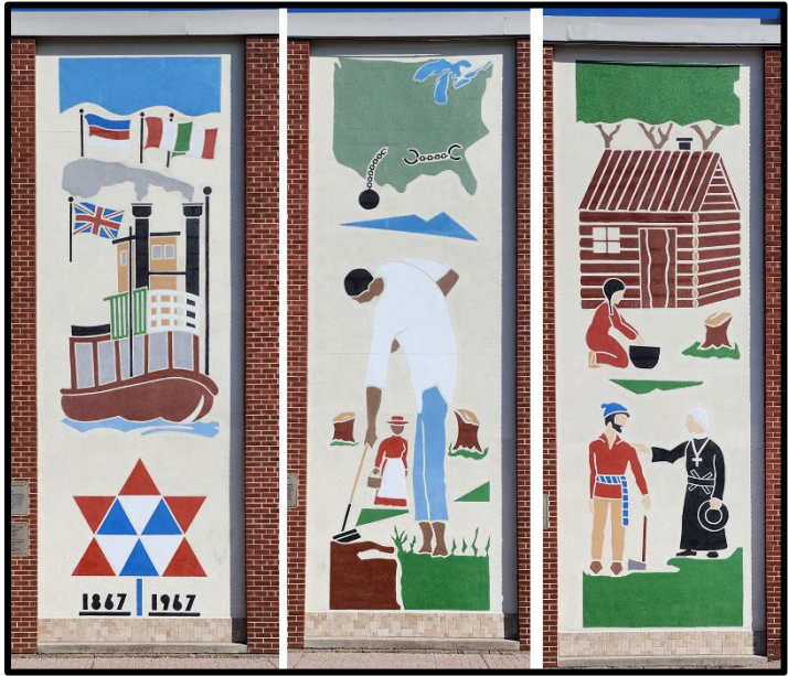
FIGURE 28 - ADDITIONAL THREE MURALS ON THE WEST ELEVATION
