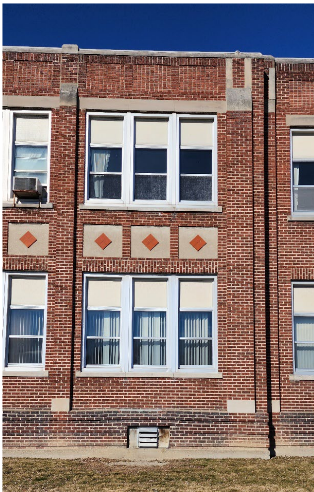
FIGURE 14 - SOUTH FACADE - WEST FLANKING BAY
