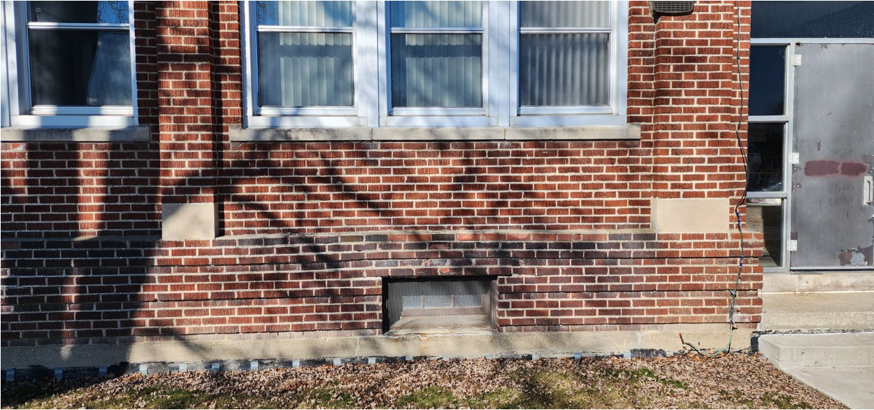
FIGURE 26 - BRICK BASE COURSING AND BANDING
