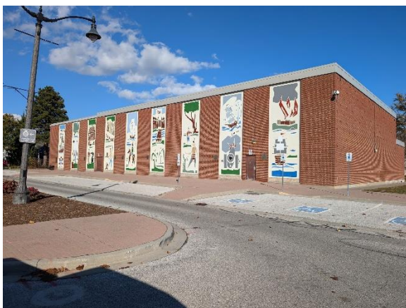
Fig. 17: West Elevation mural panels.
