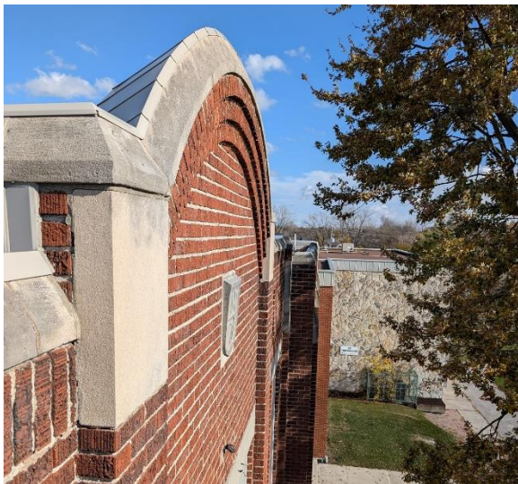
Fig. 13: Arched central bay of parapet.
