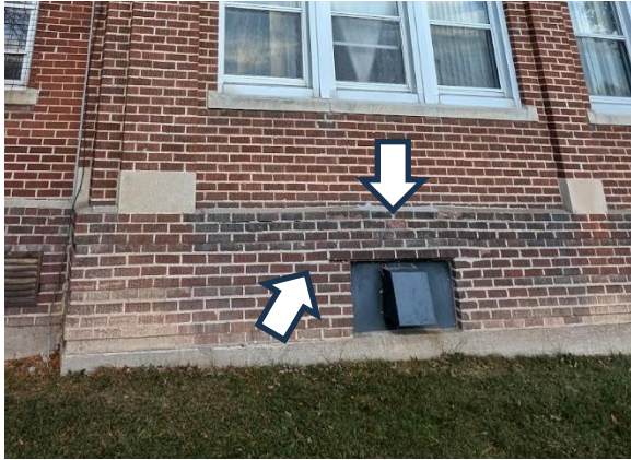
Fig. 9: Cracks, repairs to water table at base of wall
