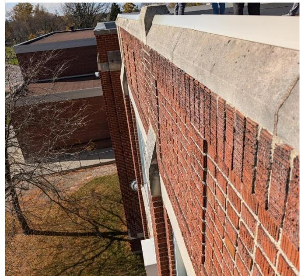
Fig. 14: Typical condition along parapet.
