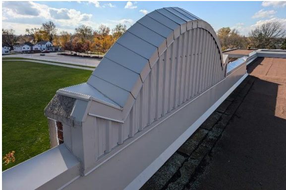
Fig. 11: Cap flashing atop parapet coping stones.
