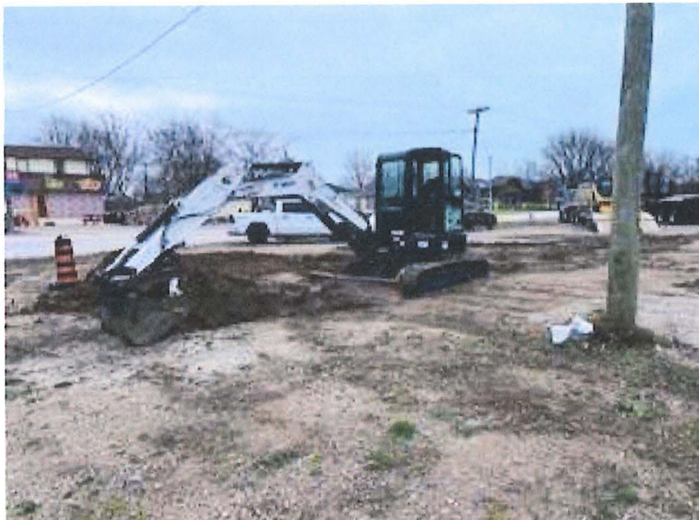
PHOTO 2 – EXCAVATION OF TEST PITS IN THE AREA OF THE EXISTING CONCRETE PAD – EAST
