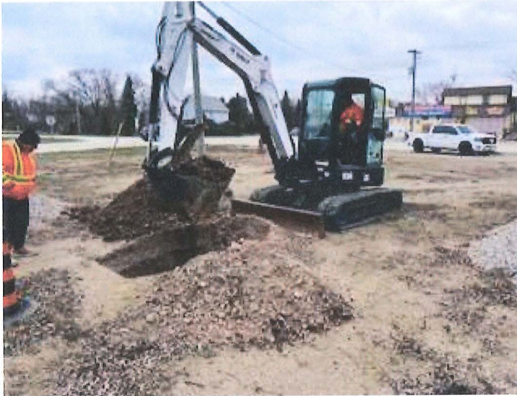
PHOTO 2 – EXCAVATION OF TEST PITS IN THE AREA OF THE EXISTING CONCRETE PAD – EAST
