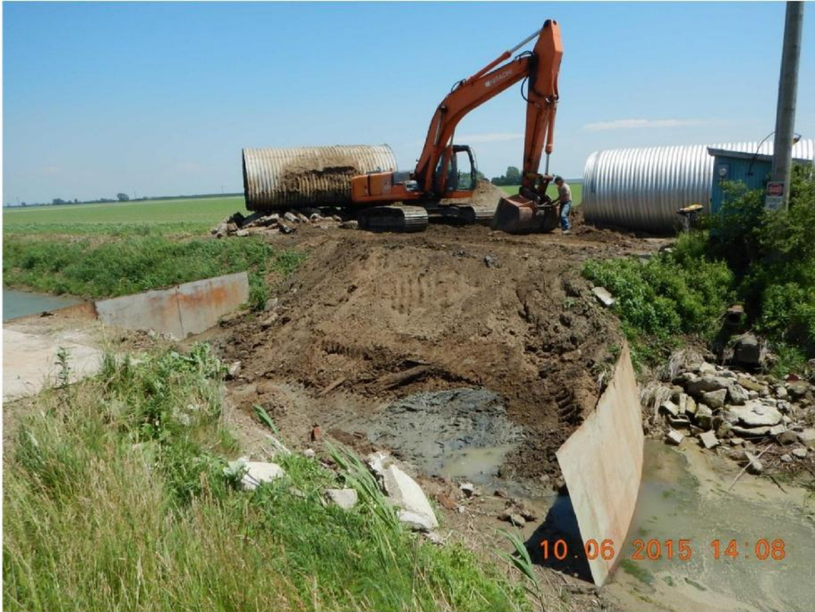
Figure 2. Isolation of Site
