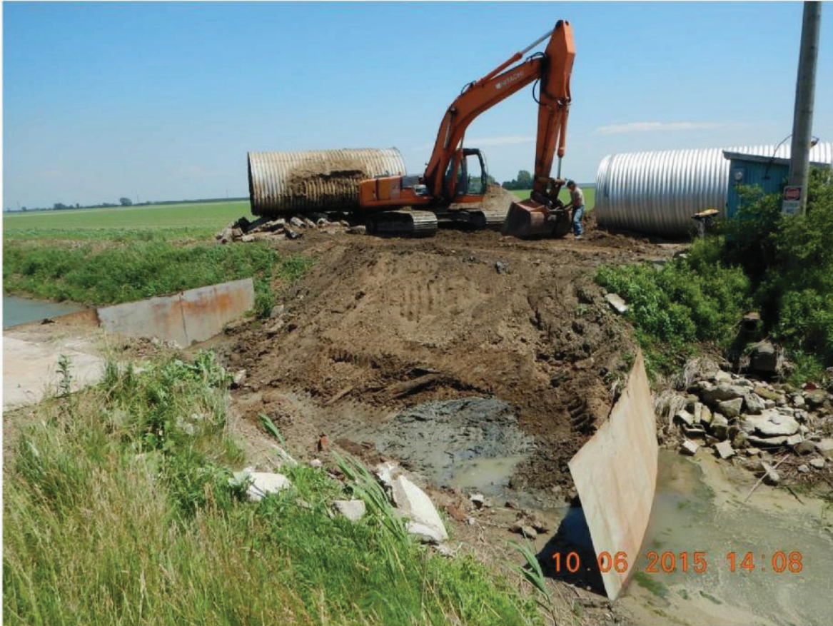
Figure 2. Isolation of Site
