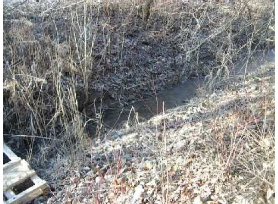
Photo 10 – Second view of ditch alongside the old rail line. At several locations there are informal trail crossings from the rail trail onto the subject property.
