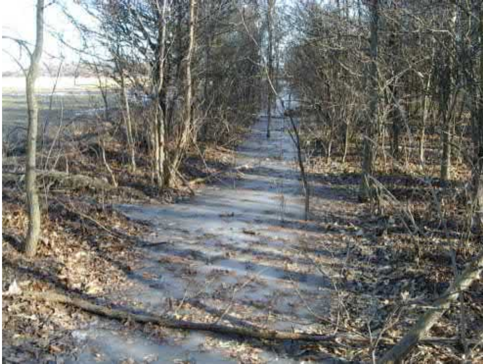
Photo 11 – View looking north along the John Knapp Drain, at the west side of the woodlot (Feature “B”). At this location, the drain is blocked with woody debris and the water has backed up. Elsewhere the John Knapp Drain is a small shallow ditch.
