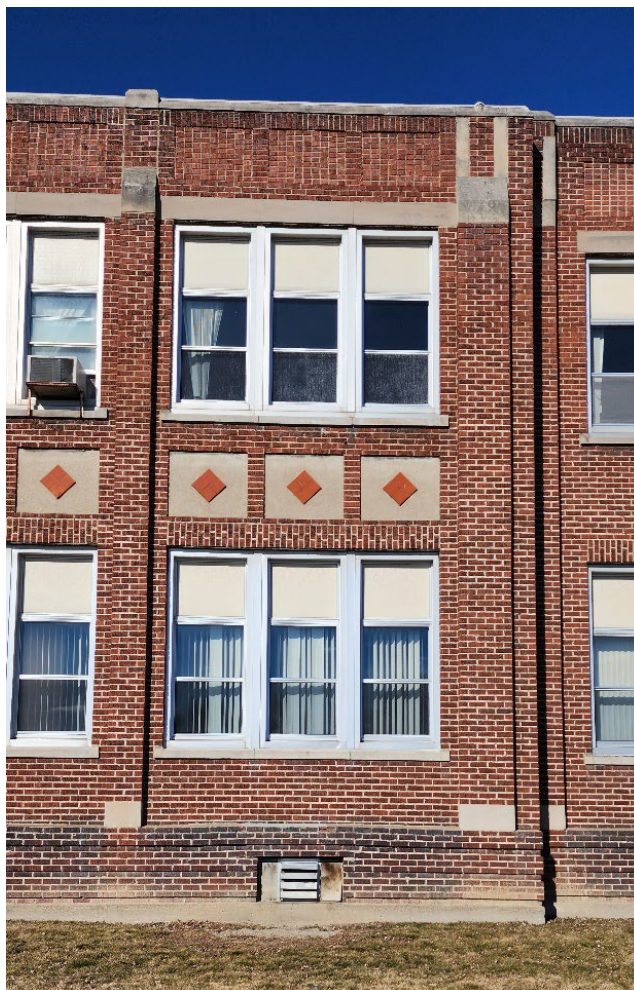
FIGURE 14 - SOUTH FACADE - WEST FLANKING BAY
