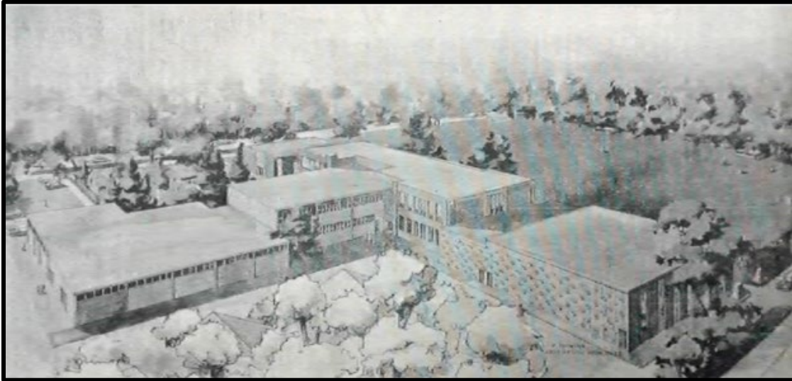
FIGURE 5 - 1964 ADDITION – THE AMHERSTBURG ECHO JANUARY 16, 1964
