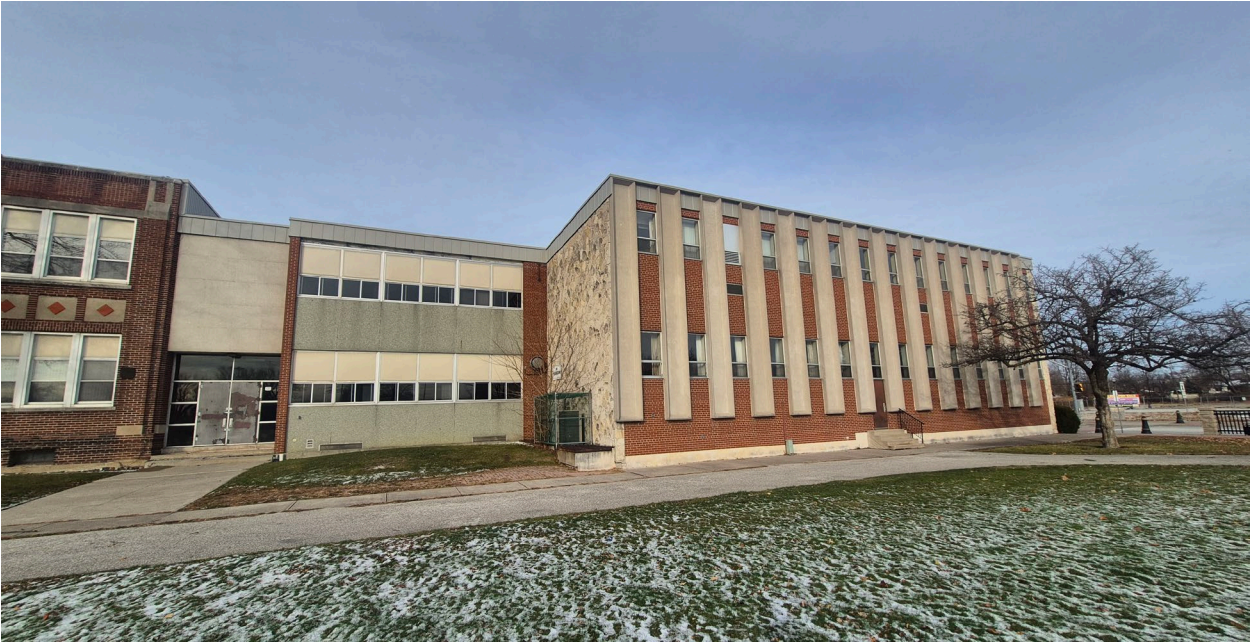
FIGURE 30 - SOUTH ELEVATION - VIEW LOOKING NORTH NEAR SANDWICH STREET
