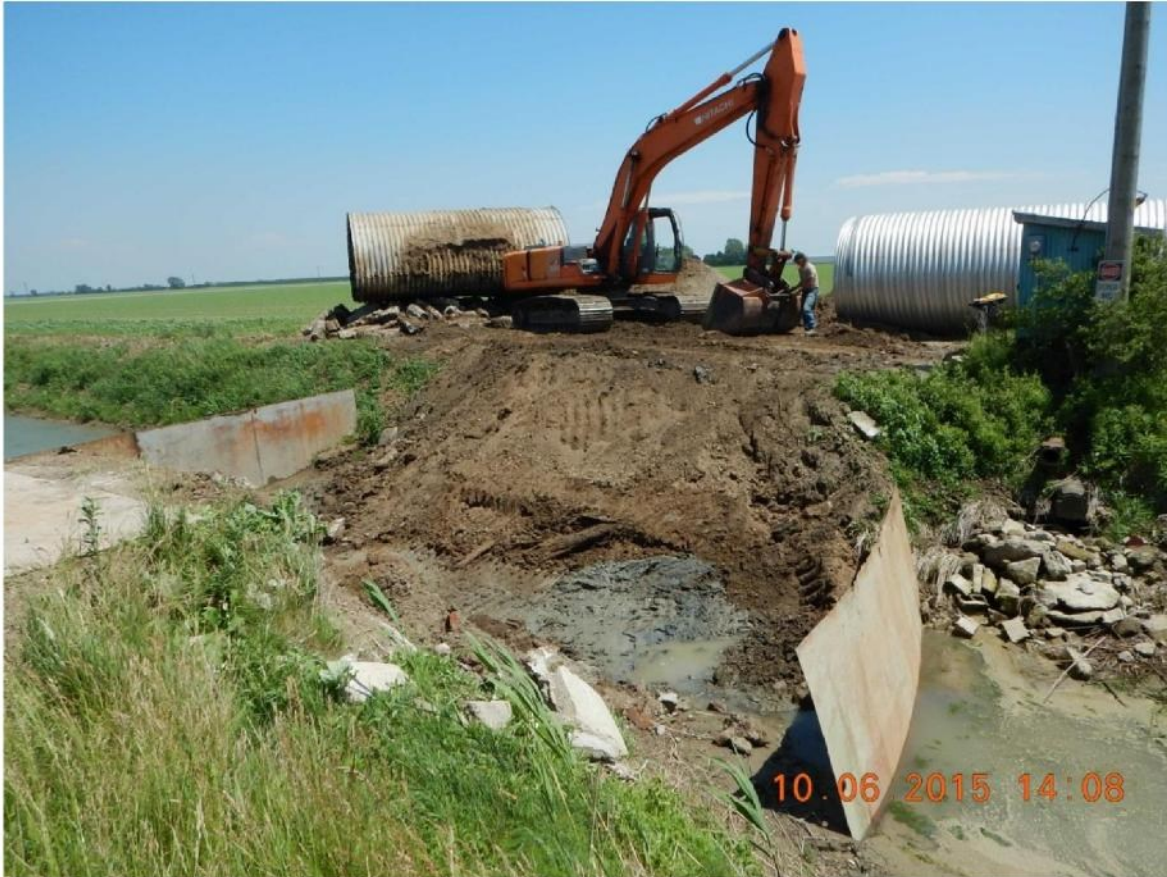
Figure 2. Isolation of Site
