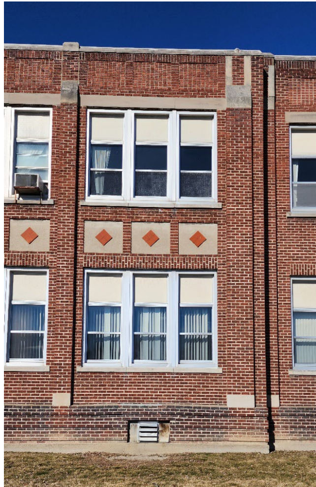
FIGURE 14 - SOUTH FACADE - WEST FLANKING BAY
