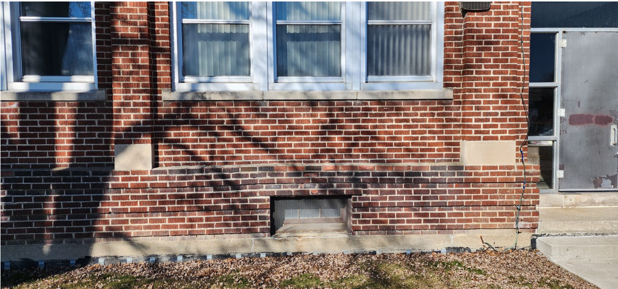
FIGURE 26 - BRICK BASE COURSING AND BANDING
