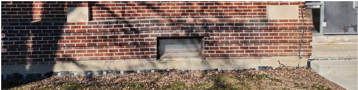
FIGURE 12 - BASE BRICK BANDING
