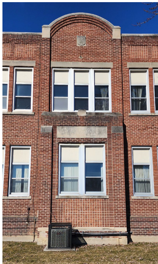
FIGURE 10 - SOUTH ENTRANCE - CENTER BAY
