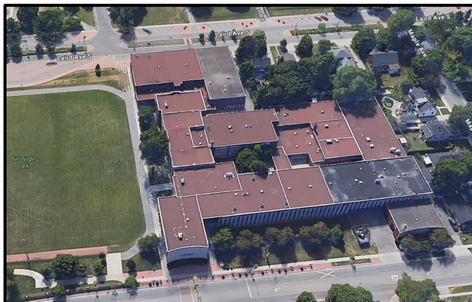
FIGURE 8 - CURRENT 130 SANDWICH ST - GOOGLE EARTH IMAGE 2025
