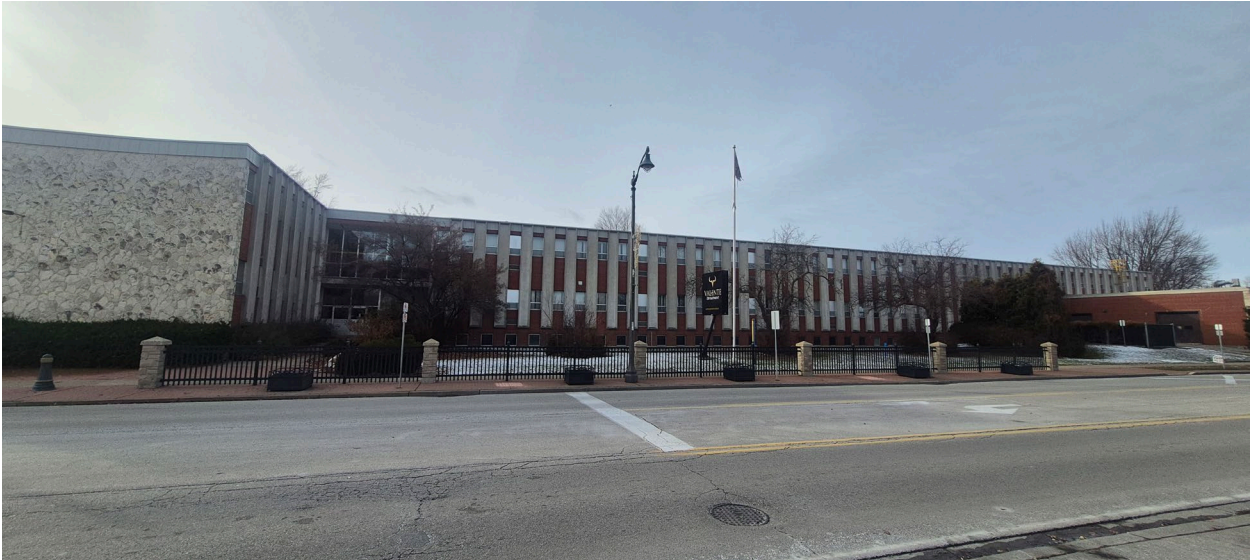
FIGURE 29 - EAST ELEVATION - VIEW LOOKING WEST FROM SANDWICH STREET.
