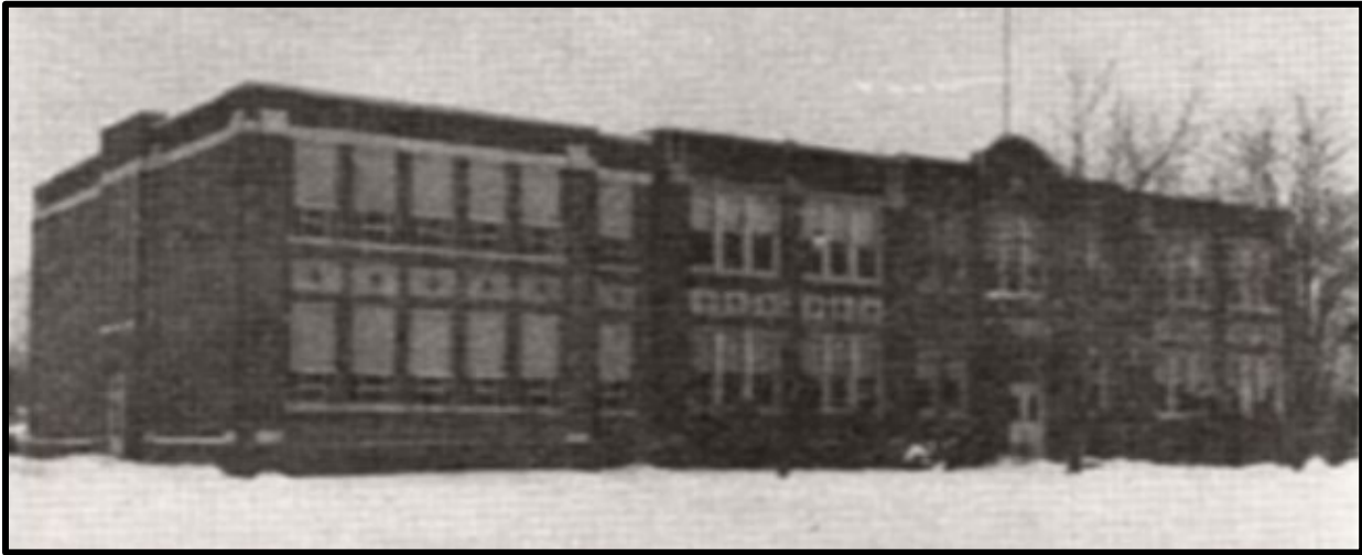
FIGURE 3 - 1951-52 ADDITION – SOURCE OFFICIAL OPENING PROGRAM
