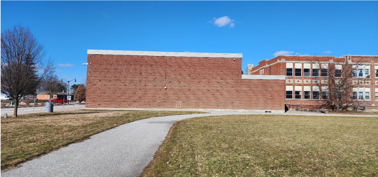
FIGURE 24 – 130 SANDWICH STREET – SOUTH ELEVATION OF GYM
