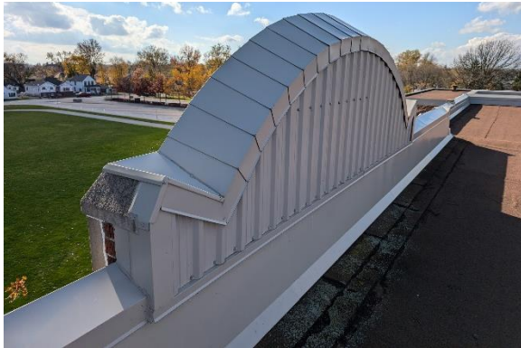
Fig. 11: Cap flashing atop parapet coping stones.
