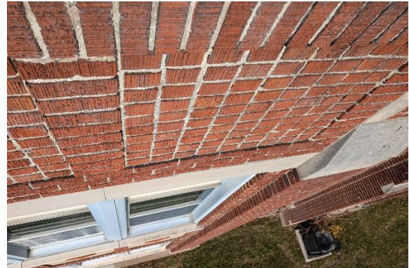
Fig. 12: Mortar joints at parapet.
