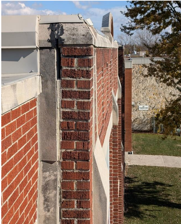
Fig. 15: Displaced stone at SW corner of facade.
