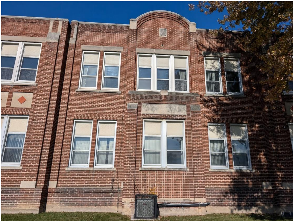
Fig 5: Closer view of façade, showing brick bond patterns, stone details, piers.
