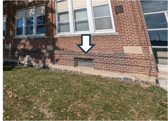
Fig. 10: Spalling brick at water table
