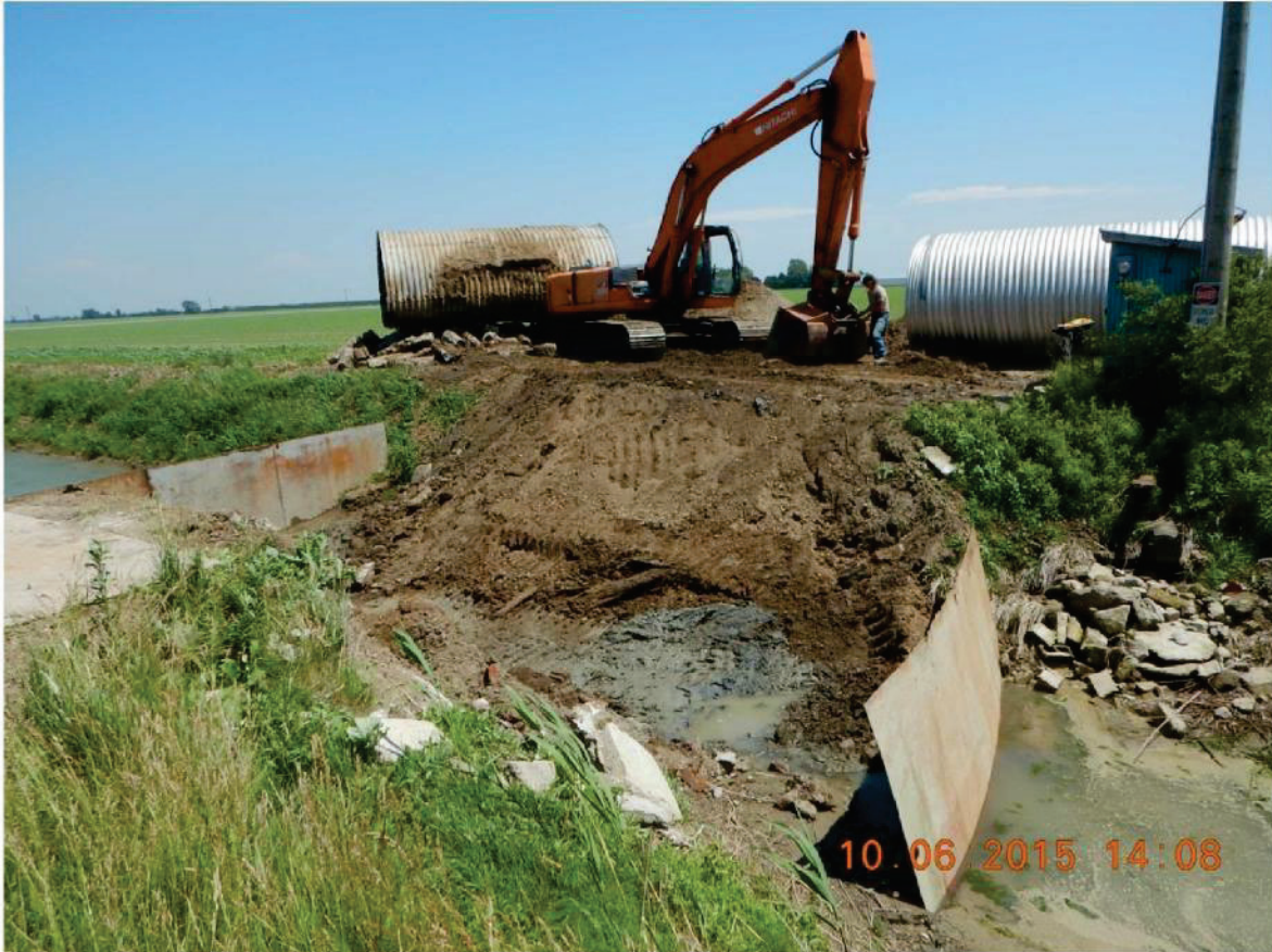
Figure 2. Isolation of Site
