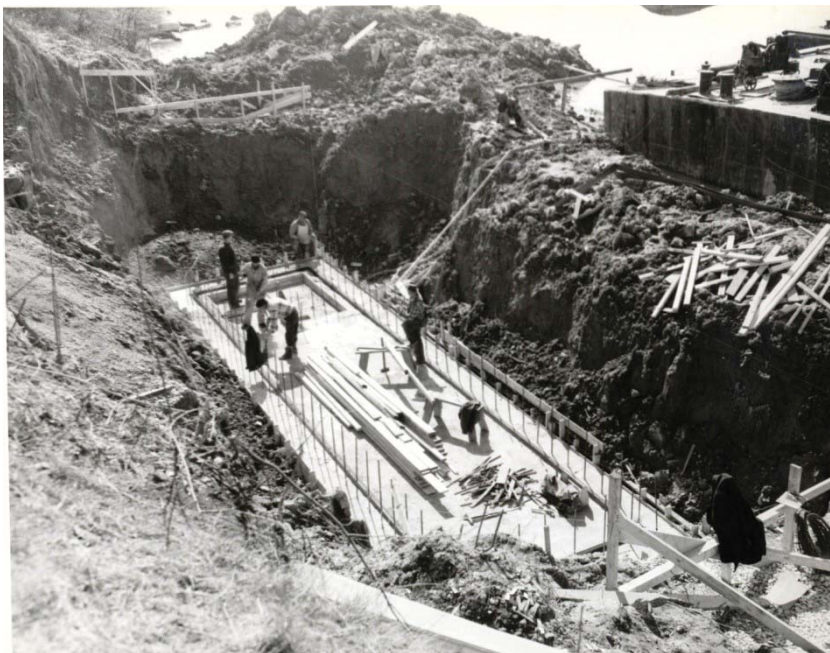
Calvert’s pump house. Foundation being built by McQueen Marine. MCS P2881.
